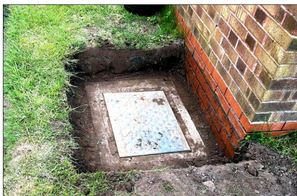
The fully uncovered manhole
